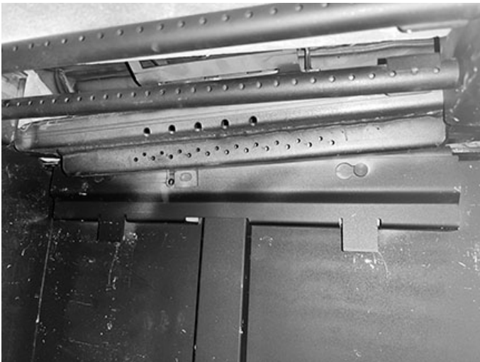
Figure 23: Remove rear baffle.
