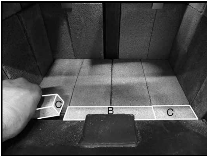
Figure 17: Narrow front bricks in place.
