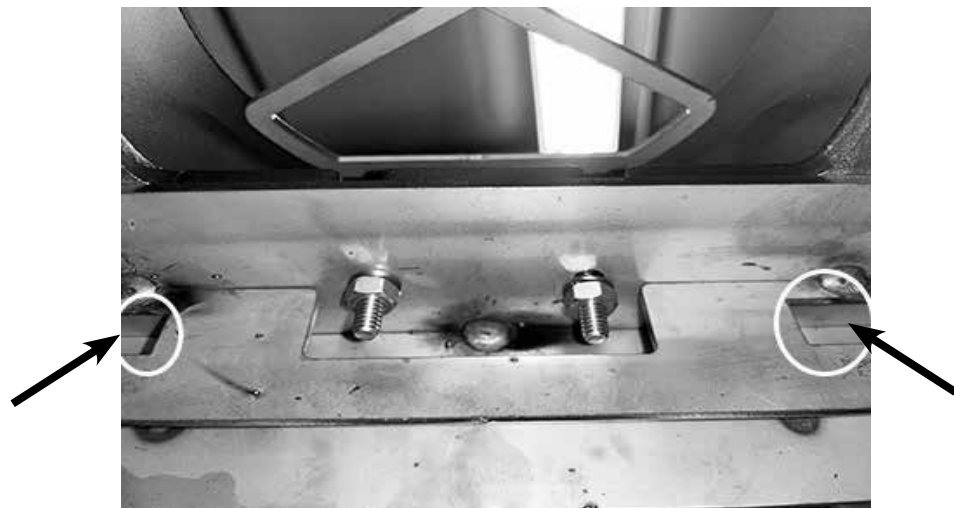
Figure 25: Front mounting slots for Flue Gas Agitator.
